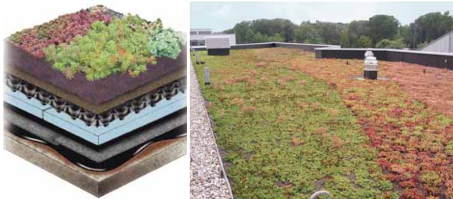
Figures 31 and 32: Green roof assembly (left), and example extensive green roof (right)
